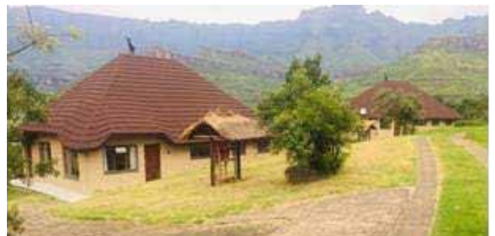
Upper Camp chalets Harvey tile installation completed.
