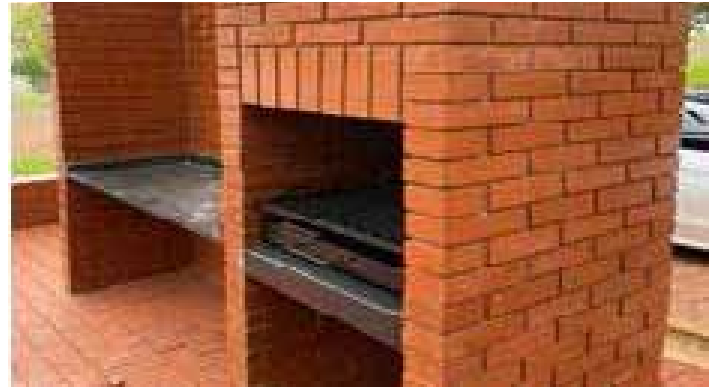
Finished structure of Braai Area
