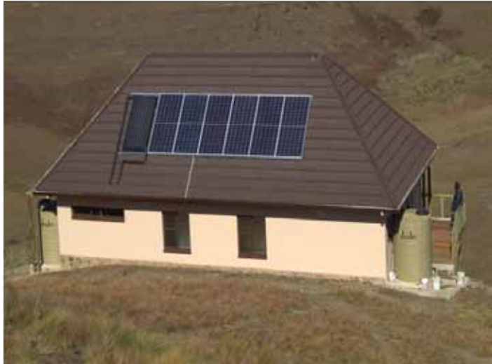
Meander Hut roof installation completed
