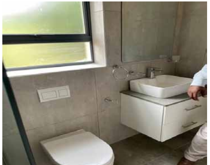
Shower and the Wall Behind the Toilet & Sink
