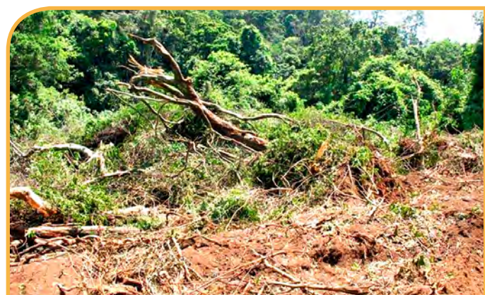
Figure 3: Unauthorised pipeline bulldozed through the Dlinza Forest Nature Reserve
